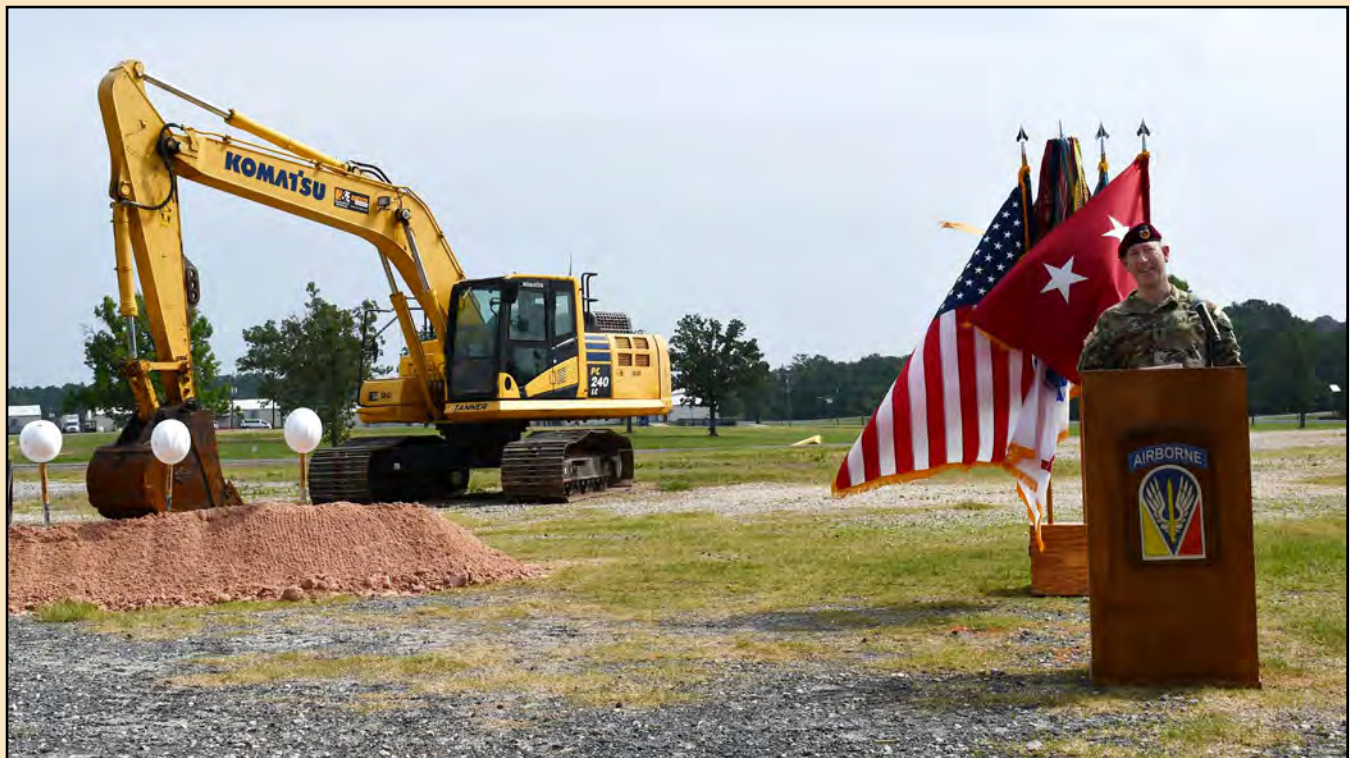
Maj. Gen. David W. Gardner, Joint Readiness Training Center and Fort Johnson commanding general, said a few words before the groundbreaking at the site of the future Joint Operations Center May 28. (U.S. Army photo by Angie Thorne)
