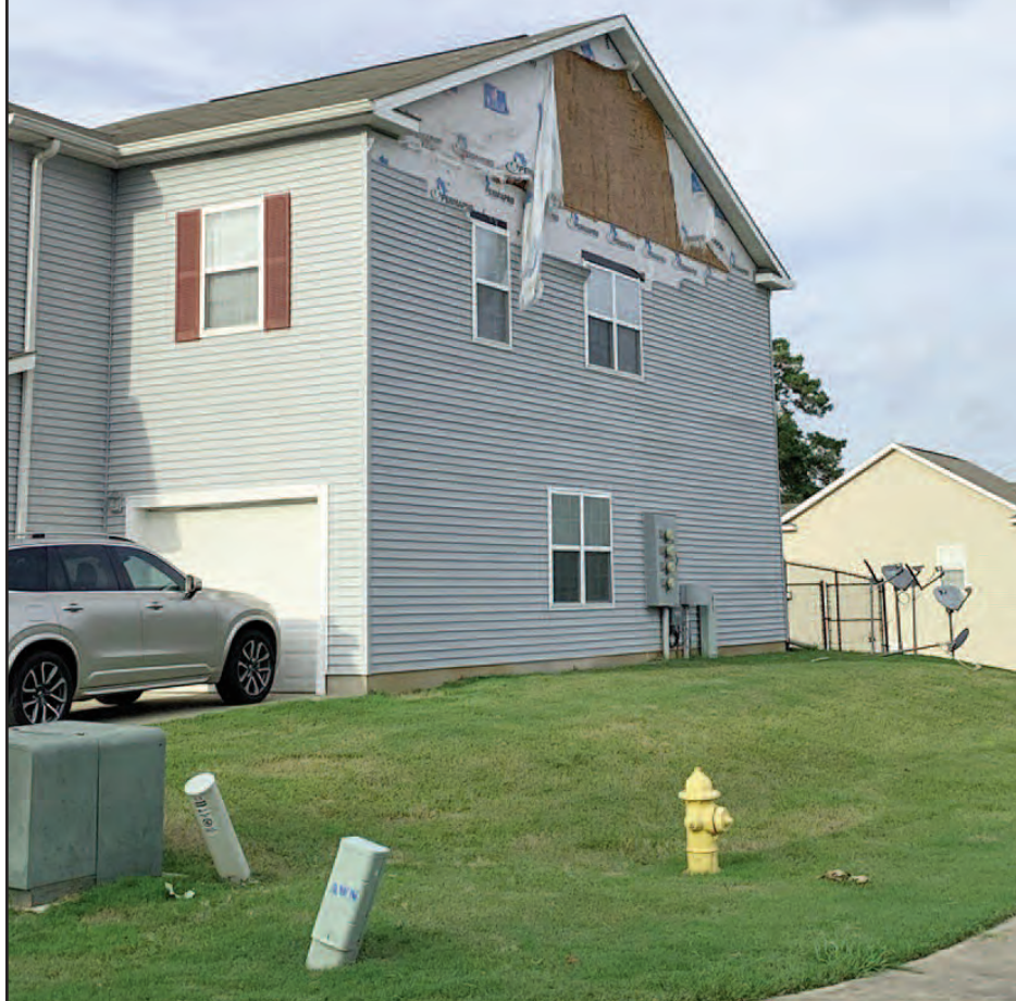
Hurricane Laura's winds ripped siding and shingles from Fort Polk housing, offices and unit buildings.
