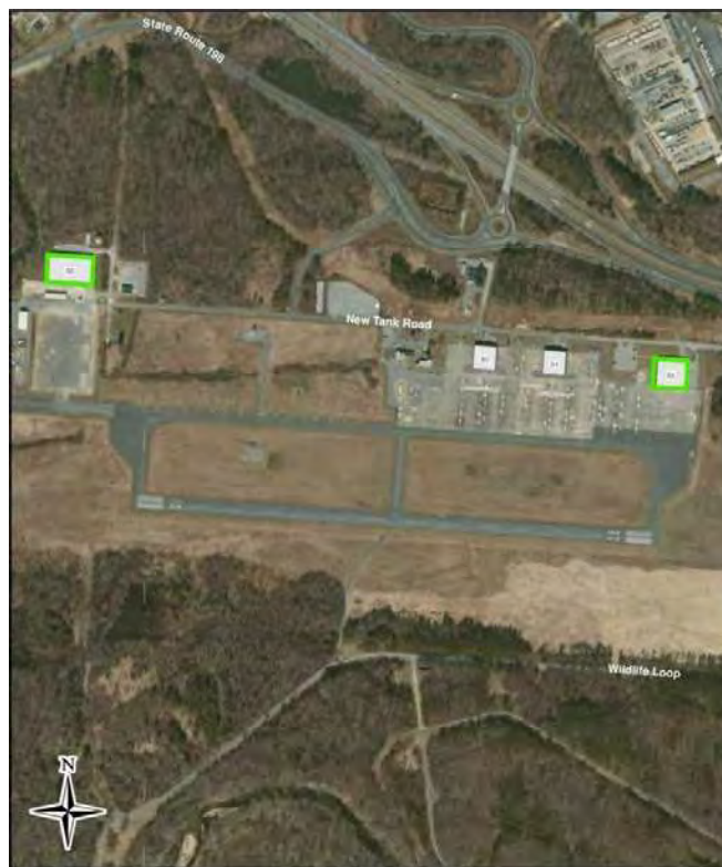
FGGM 73 (OU-28) – Maintenance Shops, Buildings 85 and 90
