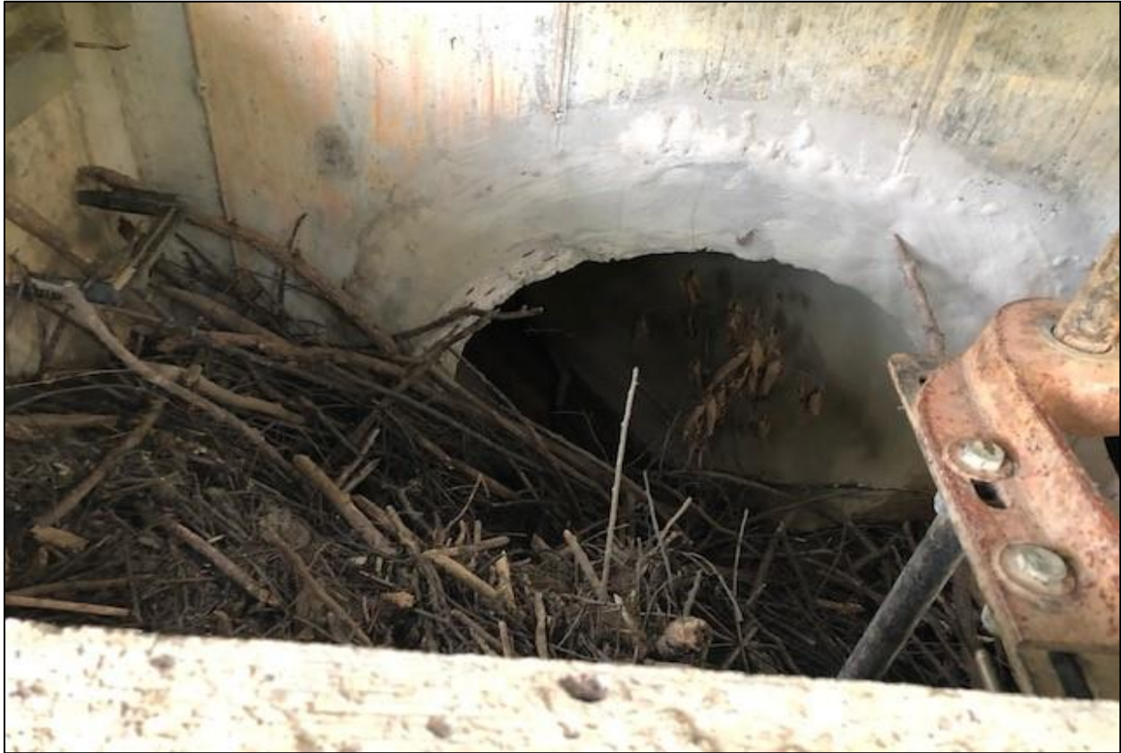
Figure 13. Evidence of Beaver Activity within the SWM Outfall Structure
