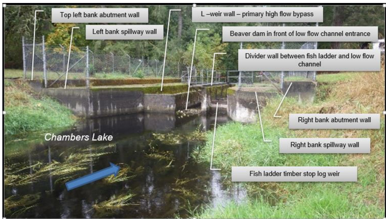
Figure 4. Chambers Lake Weir, looking downstream at inlet.
