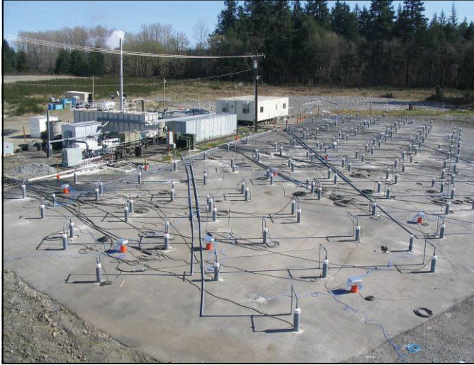
An array of electrodes produce electrical resistance heating to remove contaminants from groundwater at the Logistics Center site.
