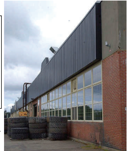
The solar heating panel on building 9580 at the Logistics Center is designed to save energy costs and help freshen the air. By Don Kramer
