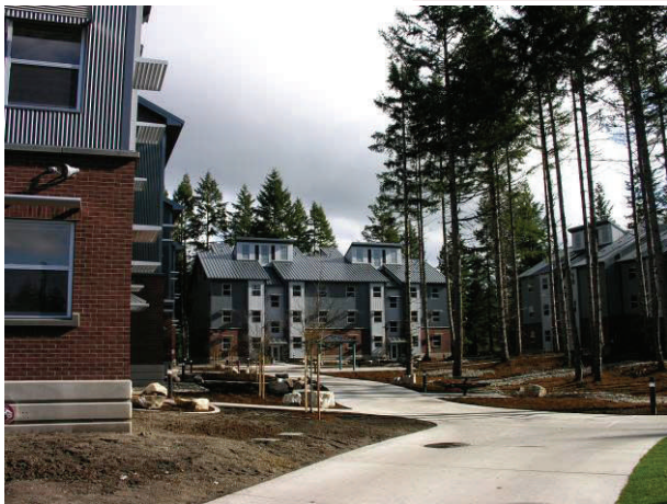
The FY 2006 Barracks complex was designed to preserve the surrounding trees, built with exterior sunshades and oriented to maximize daylighting.
