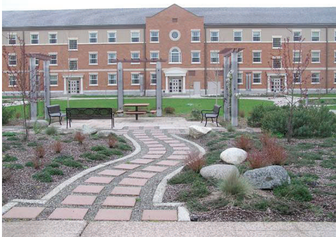
This FY 2003 Barracks courtyard features native landscaping and pavers set in pea gravel to allow storm water run-off. Photos By Jeanette Fiess, USACE
