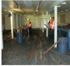
(Above) Contractors remove old growth Douglas fir flooring, historical material in the Pacific Northwest. (Left) Contractors prepare building for panelization; bringing the building down in partitions helped maximize recovery.
