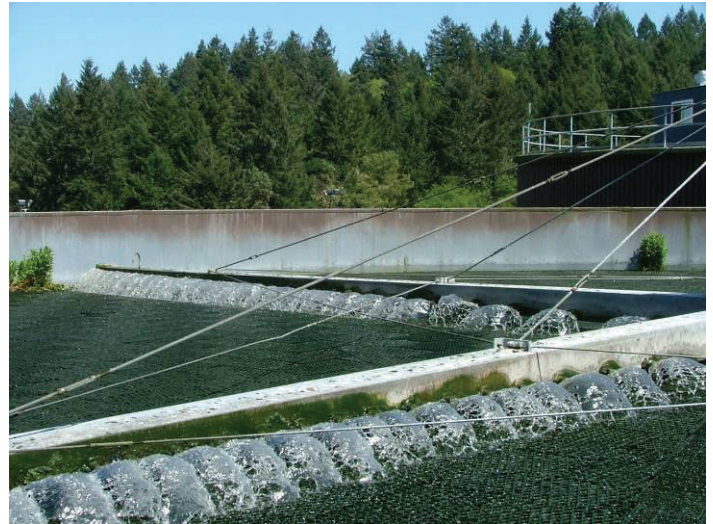
Trickling filters digest nutrients during the wastewater treatment process.
