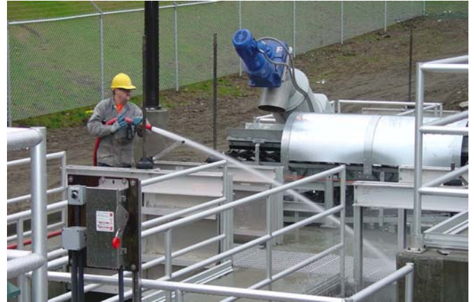
Public Works employee, Al Long, is washing down headworks equipment using treated and recycled water at the Fort Lewis Water Treatment Facility.
