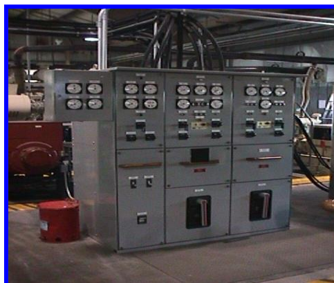
Main Switchboard Panel
