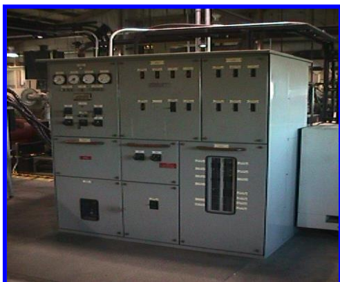
Emergency Switchboard Panel
