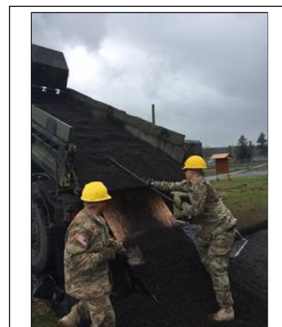
U.S. Army photo Sgt. Miguel Jaquez, left, and Pvt. Tyler Failing, right, both of the 555th Engineer Brigade, spread recycled asphalt at the Lewis Army Museum parking lot April 18, 2017.
