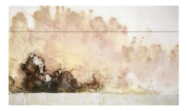
Mold growth within an occupied building is indicative of a water problem. The cause of the water problem must be investigated and resolved to prevent remediating the same site multiple times. Likewise, when water is introduced into the indoor environment the affected area must be dried as soon as possible (within 24-48 hours) to avoid the promotion of mold growth.
