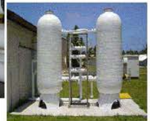
Granulated Activated Carbon Filters
