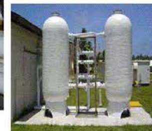
Granulated Activated Carbon Filters
