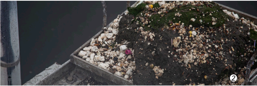
1-2) Congealed grease is removed from the wastewater supply in the early phases of the treatment process. Removal of these materials, along with foreign bodies like cloth wipes, plastics and other non-soluble solids takes a keen eye and time. Ultimately, the removal process extends the life of the island’s water pumps.
