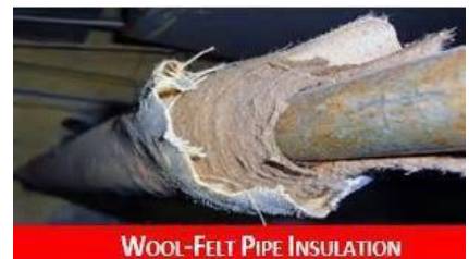
WOOL-FELT PIPE INSULATION
