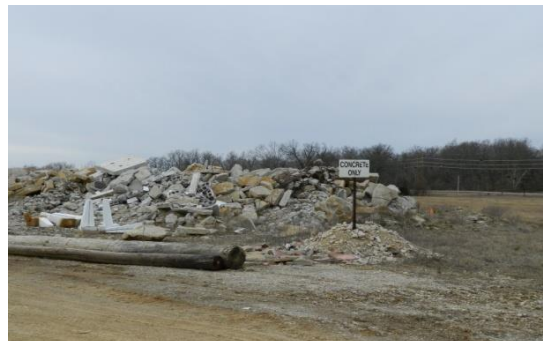
C/DD material segregated for recycling
