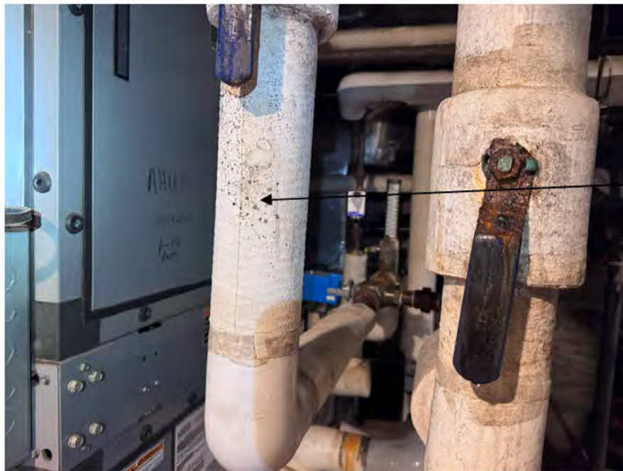
Photo 22: Mold growth observed on TSI in Basement Mech. Room 042 (Sample #M2).
