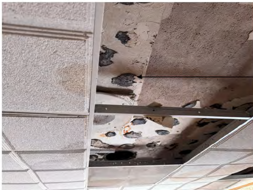
Photo 26: Brown adhesive puck associated with ceiling tile in Vestibule Room 134 (Sample #10).
