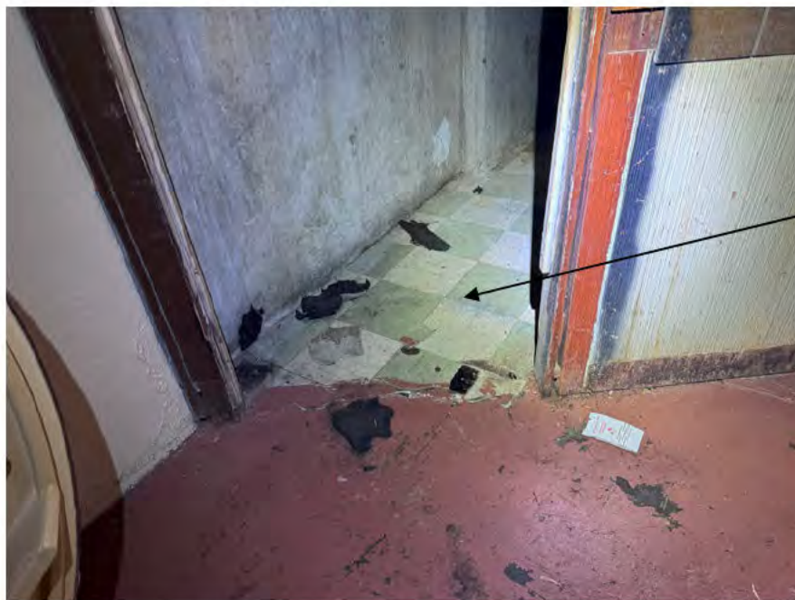
Photo 5: Two layers of ACM floor tile in Basement Room 035A (Sample #17 & 18).
