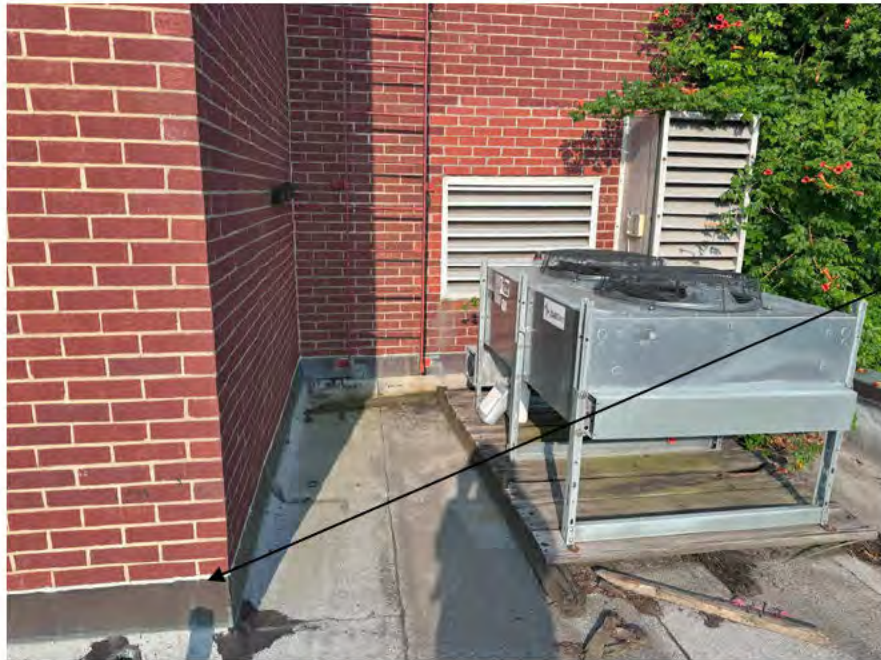
Photo 11: ACM white sealant observed on the base flashing on the roof (Sample #83).
