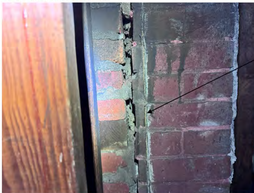
Photo 18: ACM white window frame sealant observed on a former exterior window in Mech. Room 222 and Storage Room 242 (Sample #173 & 174).
