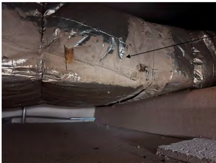
Photo 6: Yellow mastic on fiberglass insulation on HVAC duct. The yellow mastic is ACM (Sample #40).
