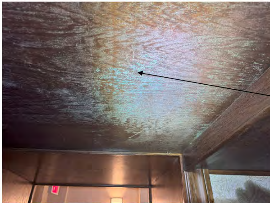
Photo 21: Mold growth observed on a wood soffit in Basement Room 055 (Sample #M1).
