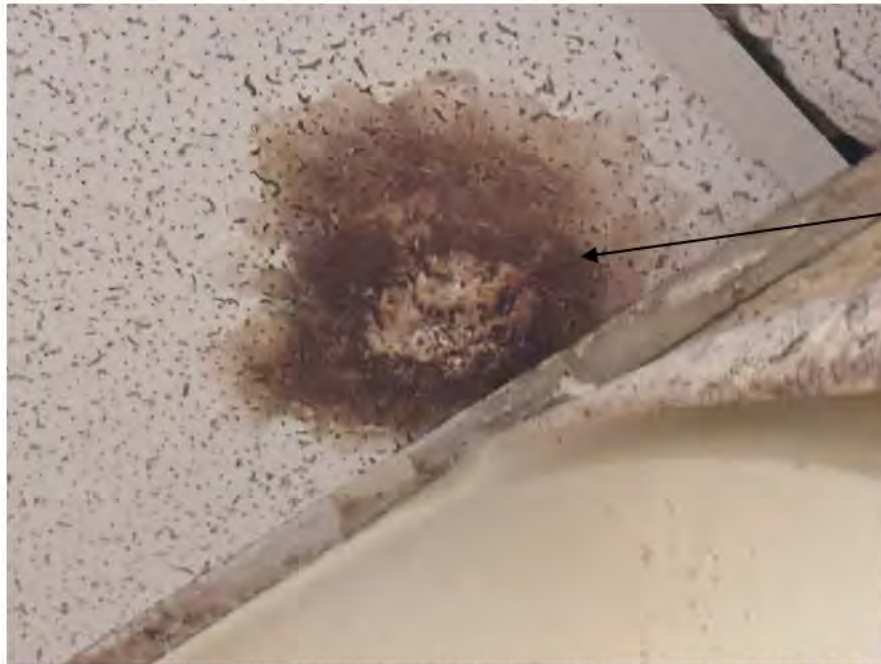
Photo 24: Mold growth observed on SACT in Kitchen Corridor 129 (Sample #M4).
