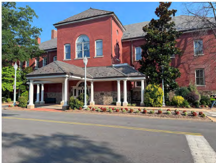
Photo 1: North facing view of the main entrance to Patton Hall, Building 214.
