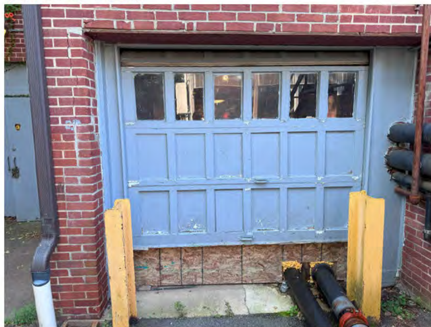
Photo 20: ACM white sealant was observed around the door frame (Sample #190).
