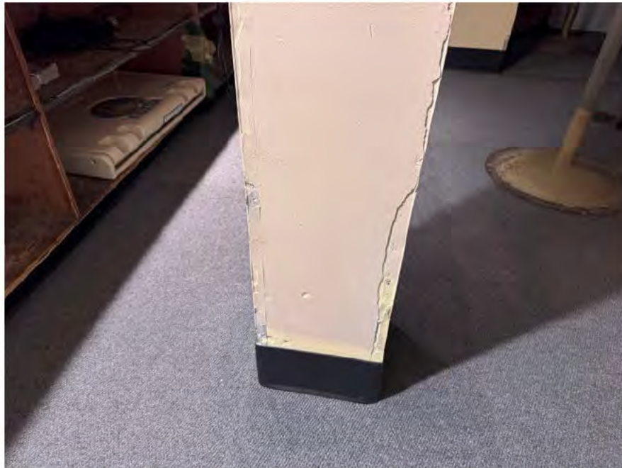
Photo 13: Gypsum wallboard and joint compound observed in Coat Room 151. The joint compound contains <1% asbestos (Sample #103).
