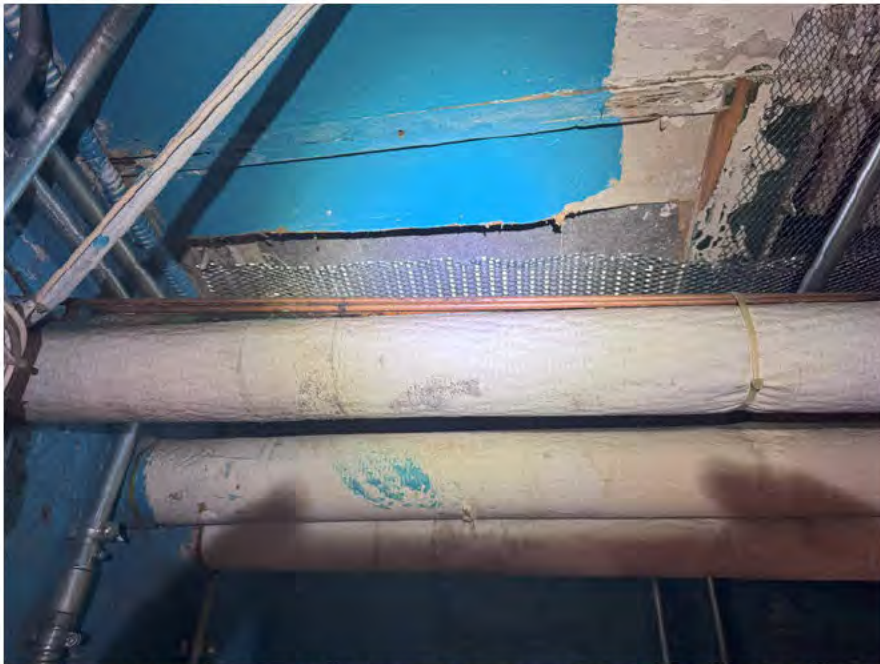
Photo 8: ACM Transite panel observed on the ceiling in Basement Mech. Room 004.
