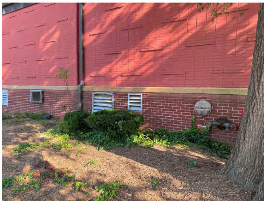
Photo 16: Exterior vents on the building. The white sealant on the vents is ACM (Sample #154).
