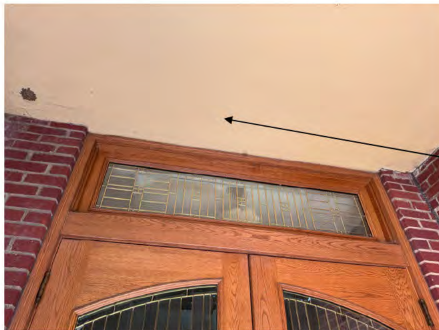
Photo 19: ACM plaster ceiling observed above the entrance to Room 134 (Sample #187 & #188).
