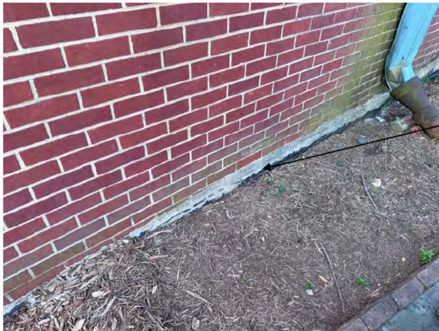
Photo 3: ACM black mastic observed at the base of the brick wall around the building (Sample #7).
