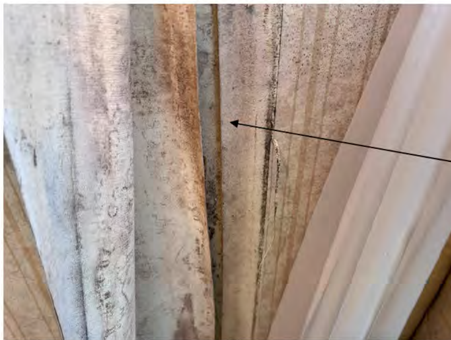
Photo 25: Mold growth observed on the backside of wallpaper in Corridor Room 228 (Sample #M5).
