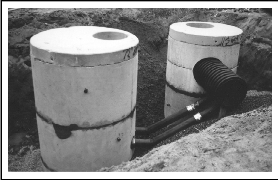
Figure 5.1: BaySeparator™ Installation at a Typical Site
