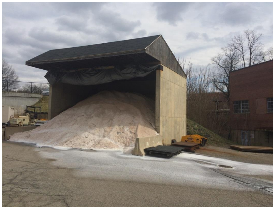
Figure 1: Improper Salt Storage – Salt shed should have tarp and barriers at entrance when pile is not actively in use
