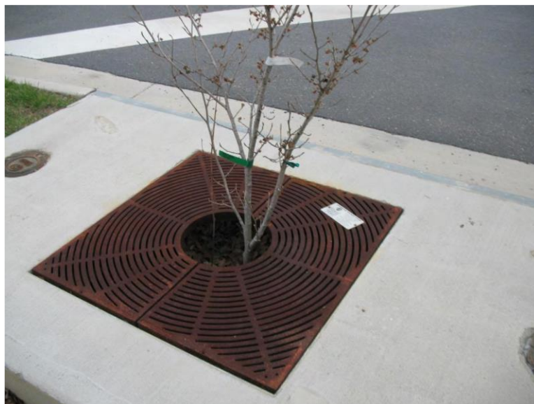
Figure 2: JBM-HH Filtterra® Unit installed at Hatfield Gate.
