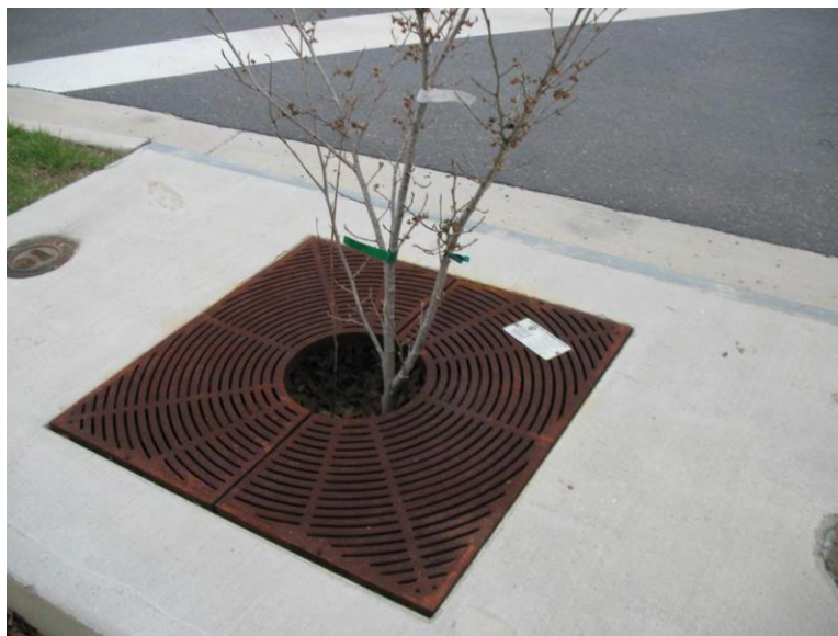
Figure 2: JBM-HH Filterra® Unit installed at Hatfield Gate.
