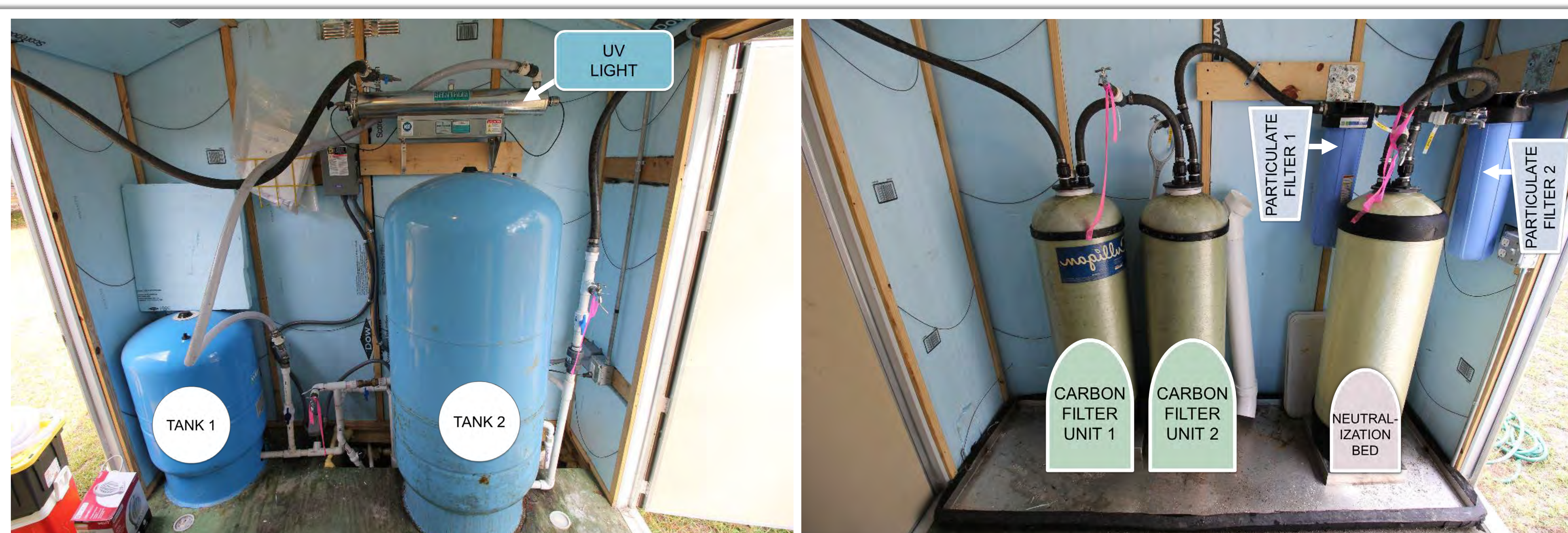
Critical Elements of the Water Treatment System, as installed
