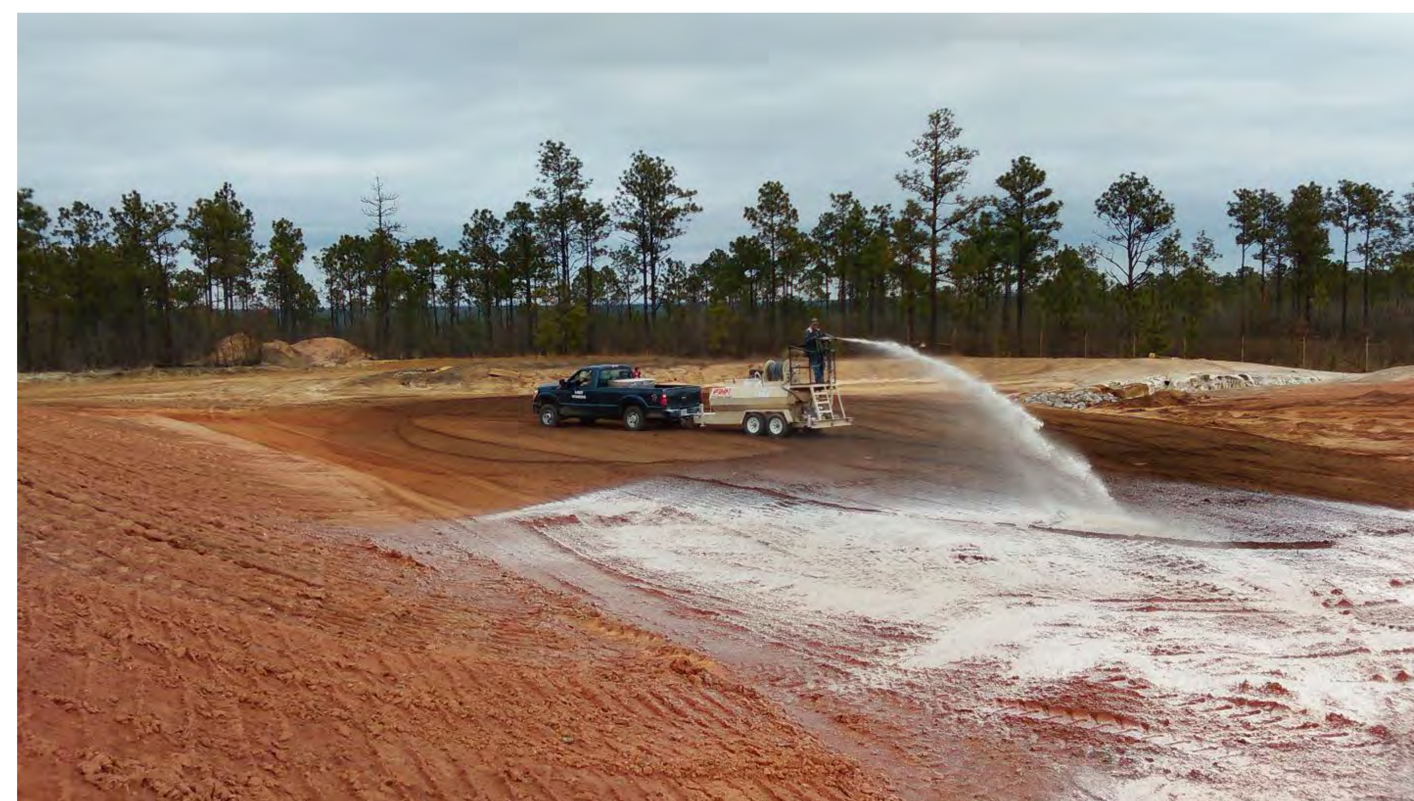
Applying lime powder to Remagen Range to raise the pH of soil and prevent explosives from getting into our groundwater
