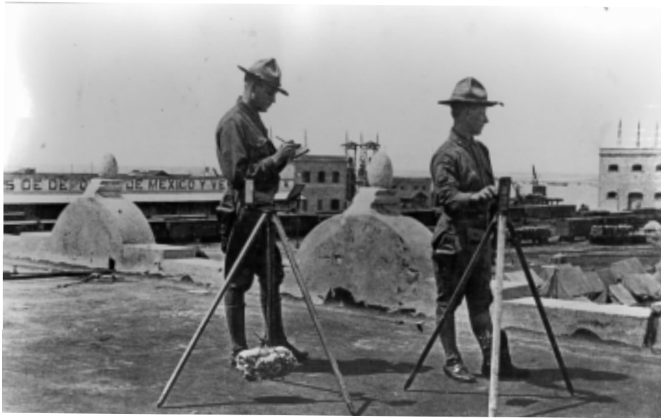
A heliograph signalling station on the roof of the Terminal Hotel, Headquarters of the U.S. Expeditionary Forces, Vera Cruz, Mexico, 1914. U.S. Army Signal Corps photo.
