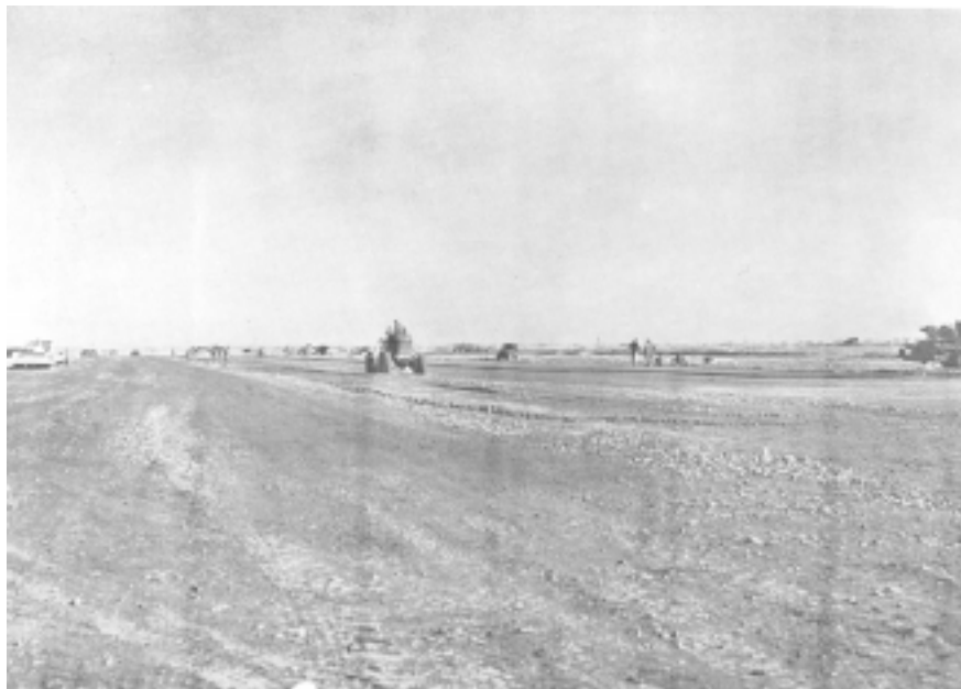
Final grading and compaction of base course in progress on runway number 2, during the construction of Libby Army Airfield at Huachuca in 1952.
