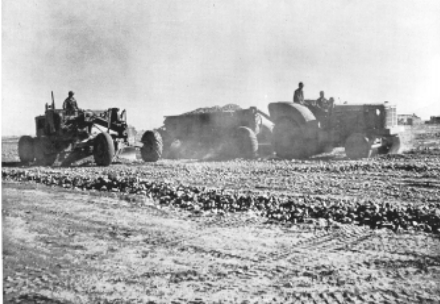
Base course material is hauled from the crusher site in dump wagons and spread by motorized graders. U.S. Army photo.
