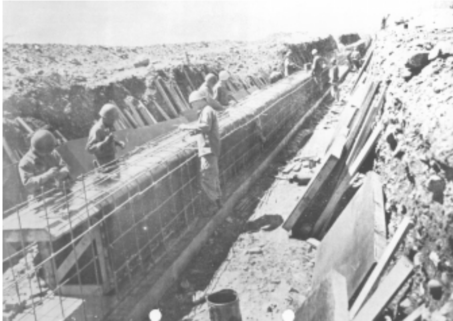
Reinforcing steel and prefabricated plywood forms are set up for a section of Culvert No. 4. U.S. Army photo.
