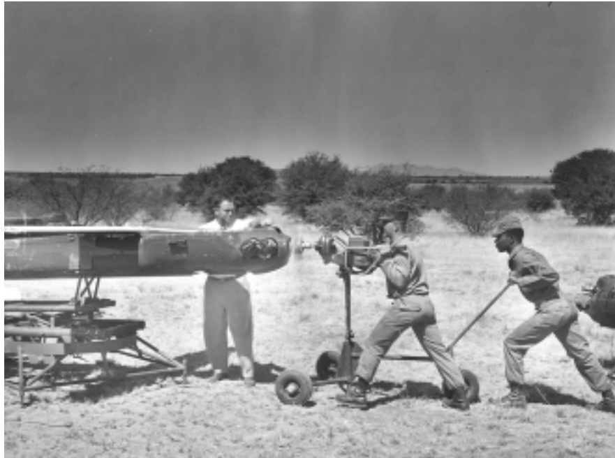
A radio controlled drone plane used for photo reconnaissance is readied for takeoff by starting crew at Fort Huachuca's USAEPG in the 1960s. U.S. Army photo.
