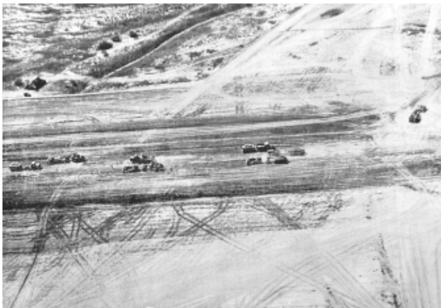
Aerial view of grading operations on runway number 2. Note use of nine separate items of engineer equipment. Work was done during the construction of Libby Army Airfield at Huachuca in 1952.
