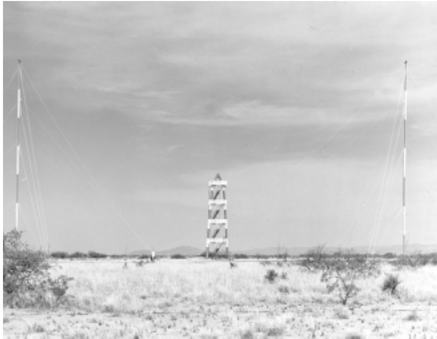
A 117-foot, all-wooden tower and the catenary suspension system at Antenna Range Site, U.S. Army Electronic Proving Ground, Fort Huachuca. U.S. Army photo.
