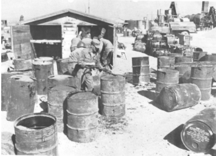
Asphalt plant personnel charge the “Hot House” during a lull in production operations. U.S. Army photo.
