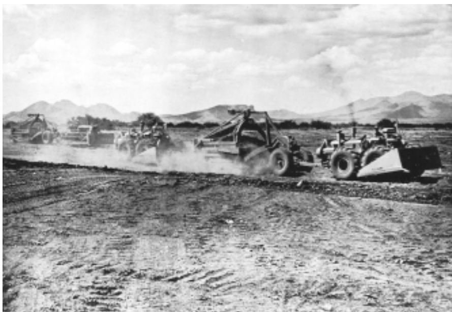
Tournadozers and towed scrapers engaged in earthmoving operations, during the construction of Libby Army Airfield at Huachuca in 1952.
