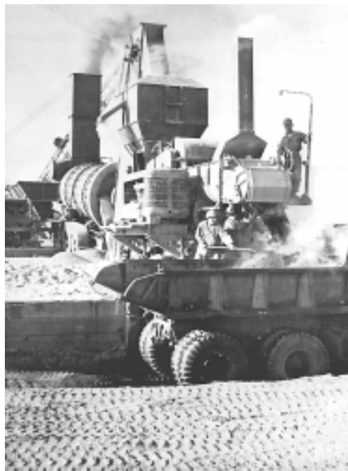
A 5-ton dump truck receives a load of hot-mix asphalt at the Paving Materials Site, during the construction of Libby Army Airfield at Fort Huachuca in 1952. U.S. Army photo.
