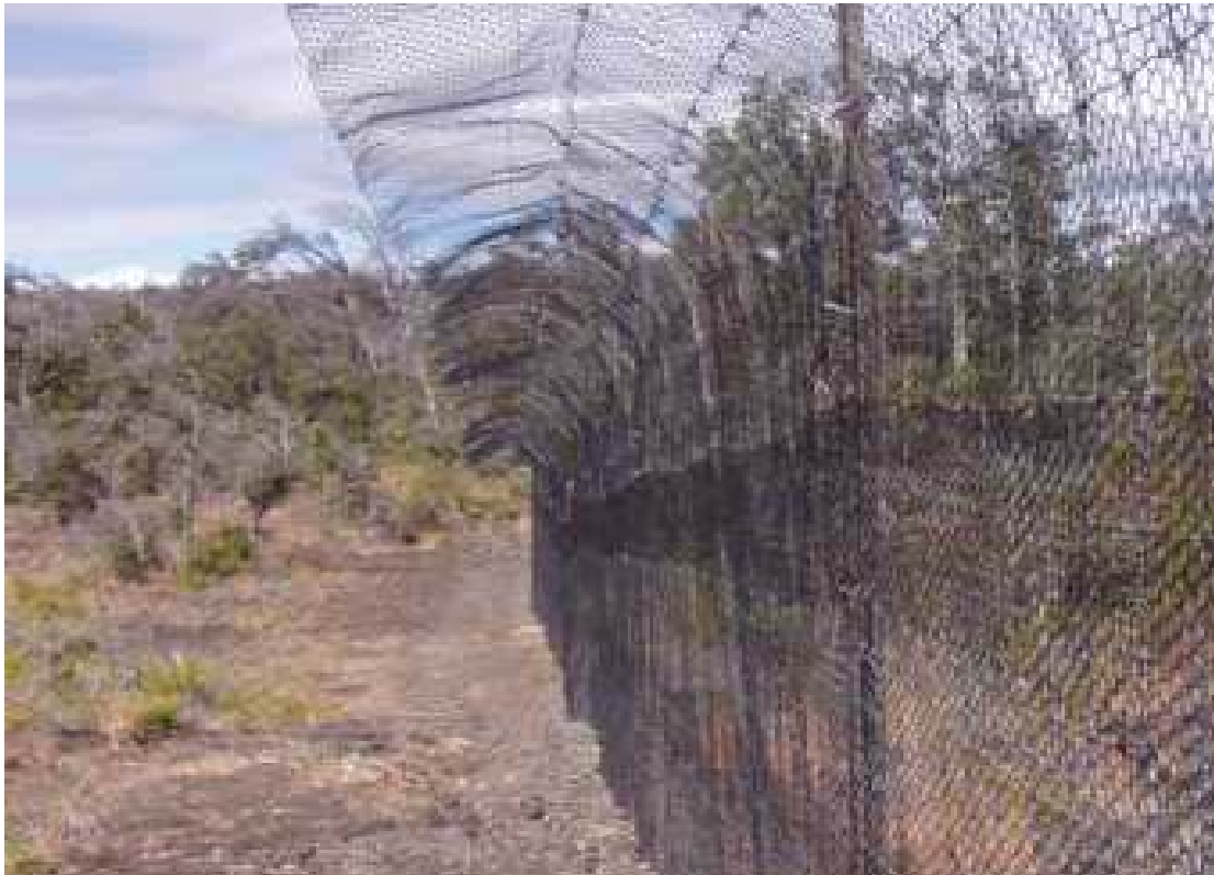
Figure 4. Example of a predator-proof fence designed to exclude cats, rats, dogs, pigs, and mongooses. The United States Army is funding construction, operation, and maintenance of two 20-acre fences for 20 years to offset impacts to Hawaiian geese at Pohakuloa Training Area by benefitting Hawaiian geese at Hakalau Forest National Wildlife Refuge.
