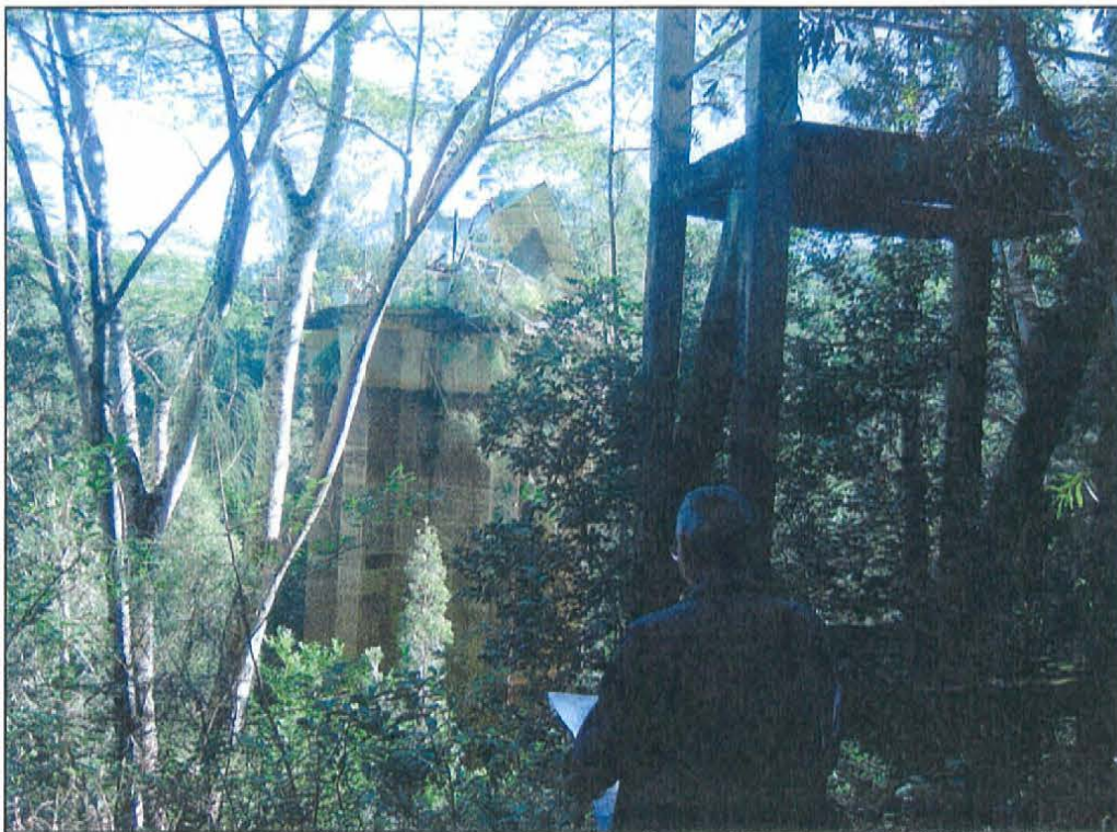
Photo 2. Top of concrete control tower and remnants of elevated access walkway.
