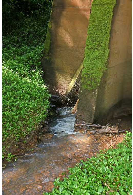
Fig. 4. Water flowing into the inlet to the drain tunnel at the base of the valve tower.
