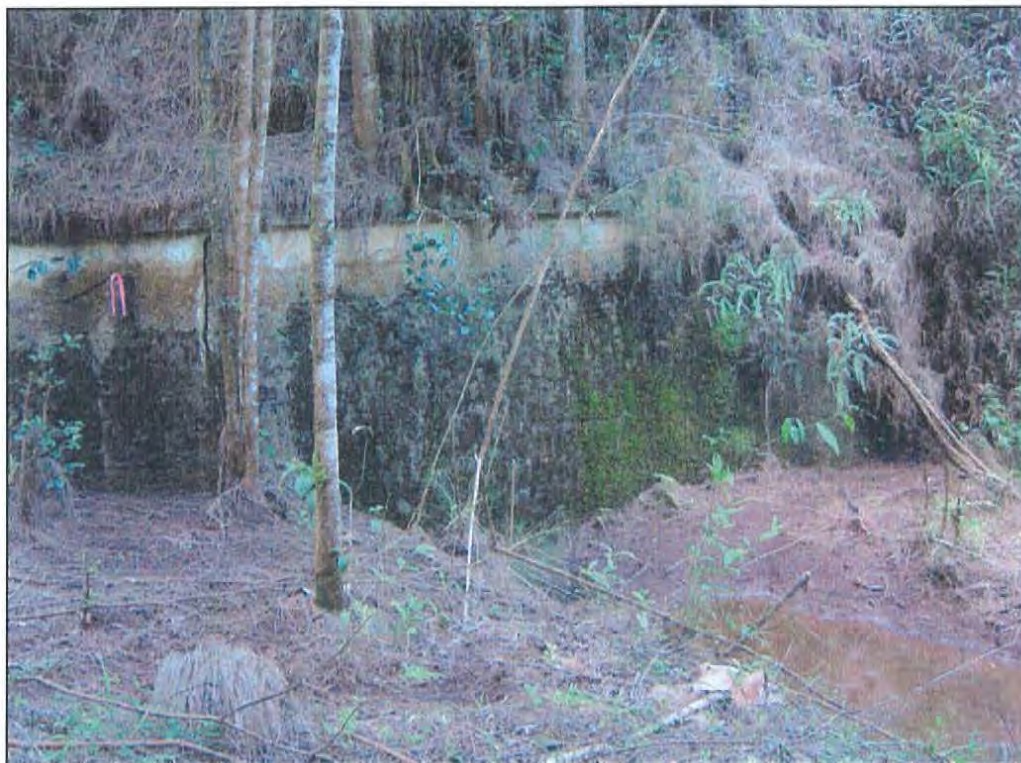
Photo 1. Concrete-lined spillway for reservoir over-flow into the natural stream channel.
