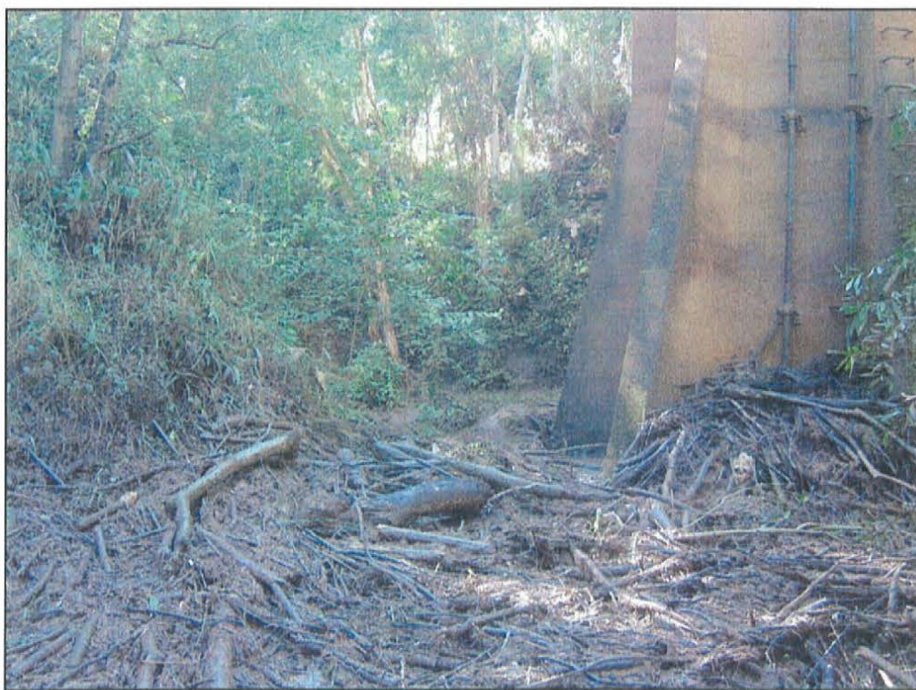
Photo 3. Tons of organic debris deposited at the control tower base after flooding.
