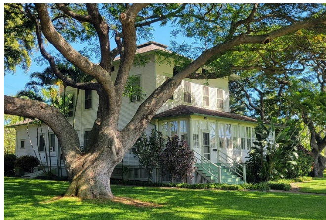
Quarters 12 at Palm Circle National Historic Landmark District.
