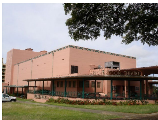
Historic Richardson Theater at Fort Shafter
