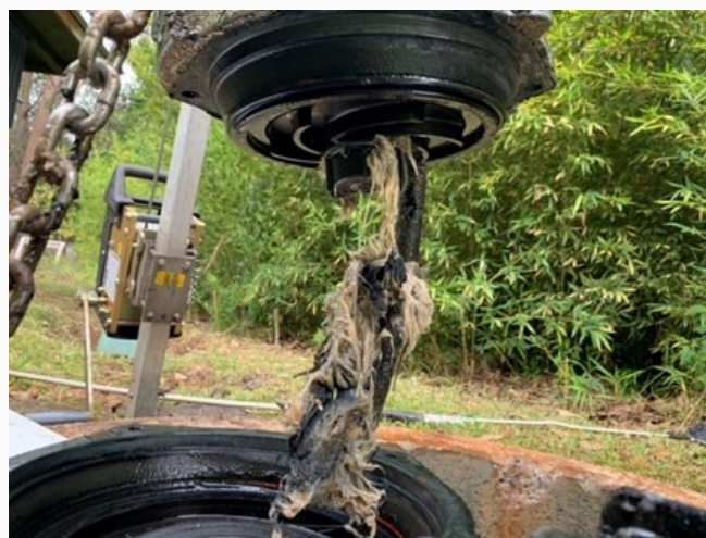
“Flushable” wet wipes caught in a pump.
