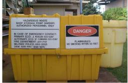
**Step 3:** Transfer the HW to the HWSSP. All drums and containers stored in the HWSSP must be marked/labeled with the words "HAZARDOUS WASTE", the name of the waste and the proper DOT hazard class.
