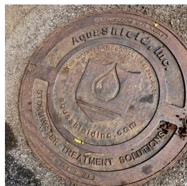
A manhole cover on a LID system.
