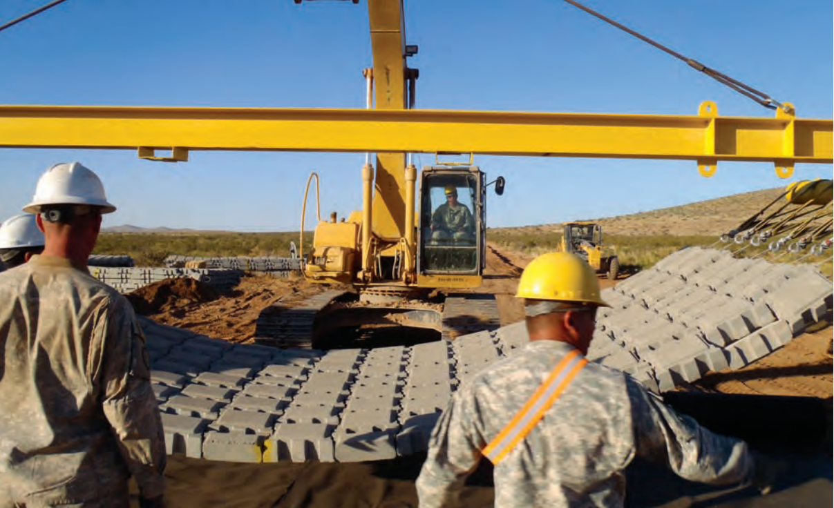
Spc. Weston Dunn, heavy equipment operator, 2nd Platoon, 561st Eng. Co., 84th Eng. Bn., 130th Eng. Bde., 8th TSC, operates a hydraulic excavator placing the Ultra Flex, an articulated concrete mat, for a low-water crossing. Staff Sgt. Albert Vila (right) controls the placement, while Sgt. 1st Class Robert Steese (left) oversees the safety of the operation, both Soldiers are with 2nd Platoon.
