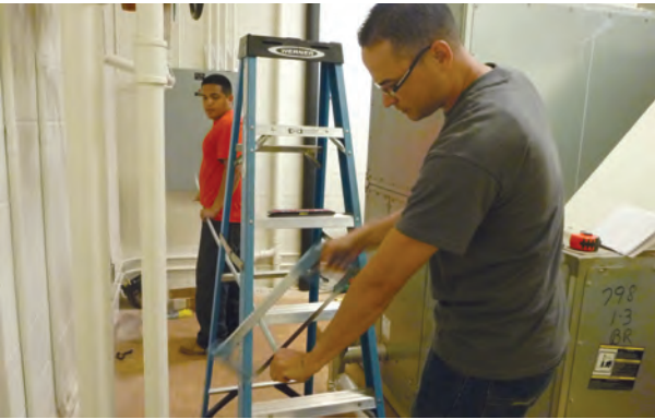
Pfc. Williams Riverasalgado (front) and Spc. Manuel Ferreira Jr. (back), both electricians with the 643rd Eng. Co., 84th Eng. Bn., 130th Eng. Bde., 8th TSC, work on cutting electrical conduits for interior lighting, as part of the DPW Trades Work Program.
