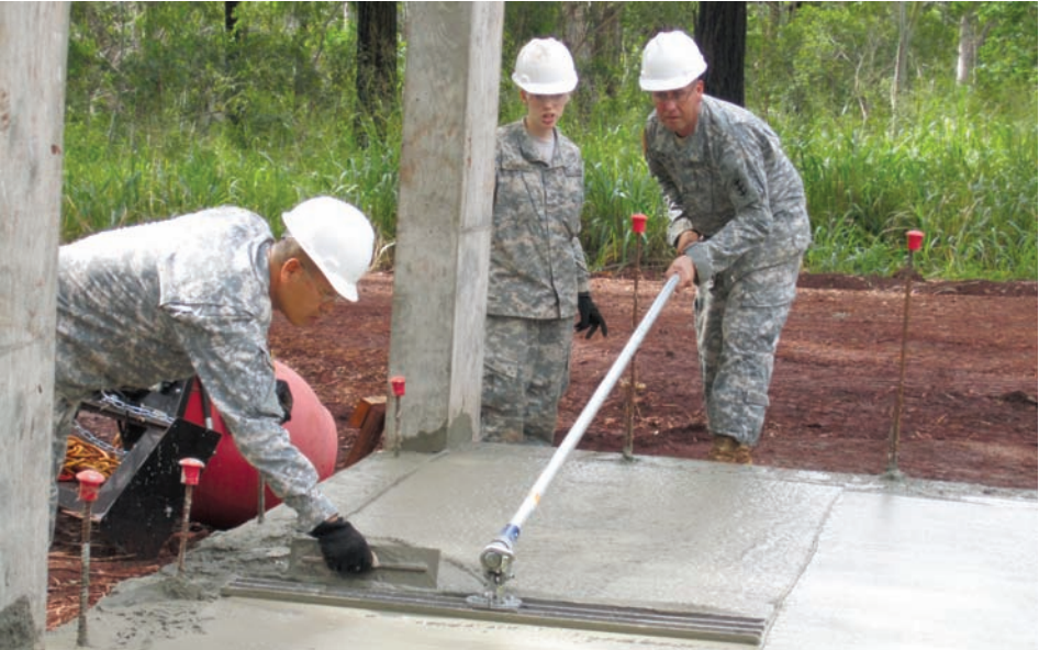
Spc. Hwan Shin (left), Pfc. Danielle Robinson (center), both carpentry and masonry specialists with the 643rd Eng. Co., 84th Eng. Bn., 130th Eng. Bde., 8th TSC, along with Sgt. 1st Class Chris Winn, platoon sergeant, 643rd Eng. Co., 84th Eng. Bn., 130th Eng. Bde., float concrete in the placement of a concrete pad, during construction of a two-room building on Schofield Barracks, Feb. 24.
