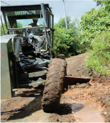
Spc. Vincent Procaccio, 523rd Eng. Company, 84th Eng. Bn., 130th Eng. Bde., 8th TSC, cleans out a drainage ditch while constructing a 1,500-meter stretch of road at the Melekeok Road Project site in Palau, recently.
