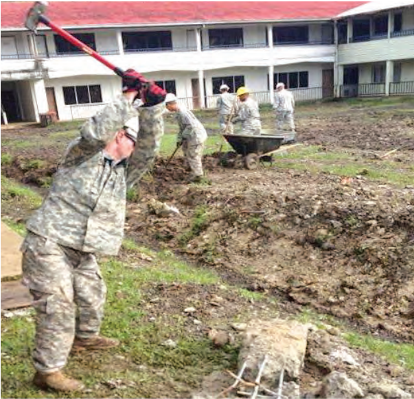
Soldiers from Construction Civic Action Detail break through old, reinforced concrete at an elementary school in Malem Village during a ditch-draining project as part of the company's four-month deployment.
