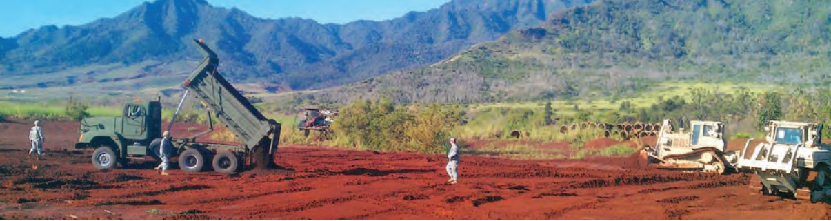
Soldiers from 2nd Plt., 523rd Eng. Co., 84th Eng. Bn., 130th Eng. Bde., 8th TSC, cut and fill the range as the 3rd Plt. “Construction Ninjas,” 523rd Eng. Co., haul in dirt.
