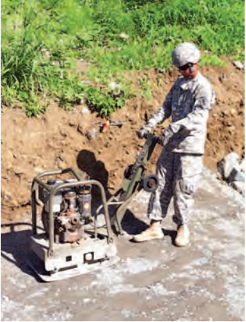
Pfc. Jose Cervantes, 1st Plt., 561st Eng. Co. (Horizontal), 84th Eng. Bn., 130th Eng. Bde., 8th TSC, uses the hand tamper to reach the necessary compaction level to install a small culvert.
