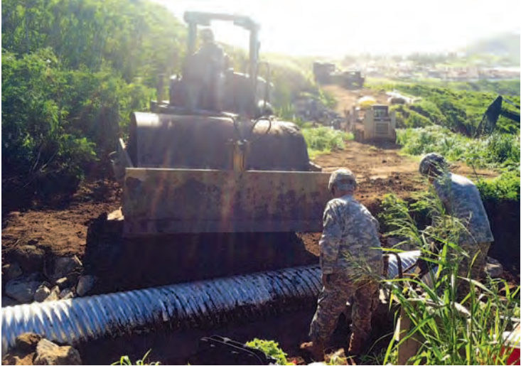
The 1st Plt., 561st Eng. Co. (Horizontal), 84th Eng. Bn., 130th Eng. Bde., 8th TSC, installs a 16-foot culvert to prevent heavy rain flow from impeding travel along a combat trail.
