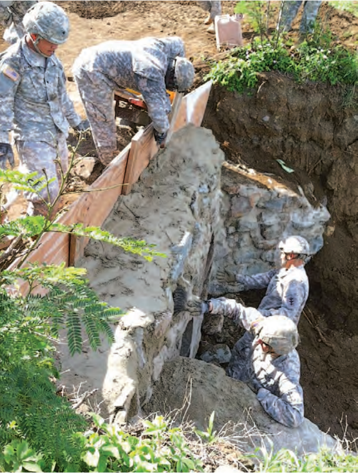
Soldiers with 3rd Plt., 643rd Eng. Co. (Vertical), 84th Eng. Bn., 130th Eng. Bde., 8th TSC, strike the joints of the headwall with mortar at a large culvert site over the holidays.
