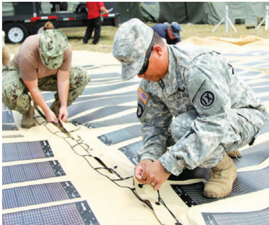
Sgt. Roy Gano (right), carpenter/masonry tech, 871st Engineer Company, 9th Mission Support Command, becket-laces a solar shade canopy during the setup of a humanitarian aid and disaster relief exercise, July 7. The solar shade has the potential to provide enough energy for several days of continuous 24-hour use.
