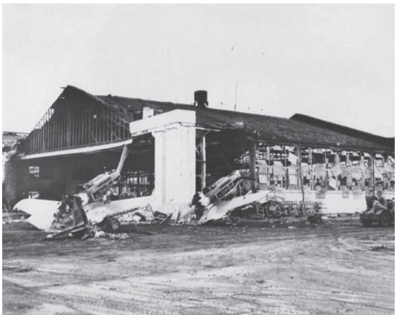
Hangar #3 and aircraft are damaged on Wheeler Field after the attacks.
