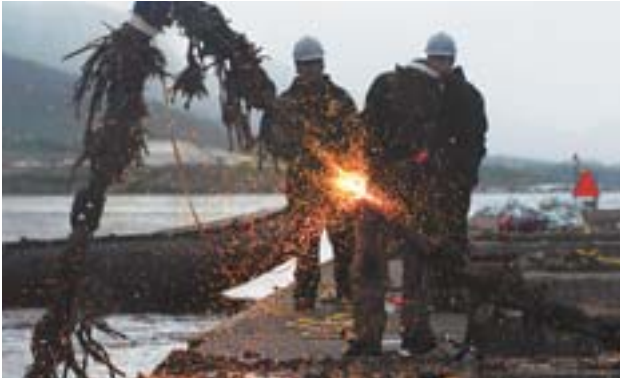
Staff Sgt. Andrew Harrison, diving supervisor, 7th Engineer Diving Team, cuts an old chain that holds the breakwater in place. The team is in Ketchikan, Alaska, repairing a floating breakwater in Bar Point Harbor.
