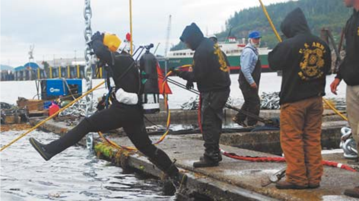
Sgt. Jake Cochran, lead diver, 7th Engineer Diving Team, leaps into Bar Point Harbor in Ketchikan, Alaska, during a breakwater improvement project. During the dive, Cochran surveyed the old chain on the sea floor and prepared it for removal.
