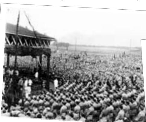
Soldiers gather at the “Boxing Bowl” for a show in 1931. The original building, now known as the Conroy Bowl, was built in 1923, and only the center stage was covered. By 1932 a roof was added. Today the building is mainly used for staging deployments.
