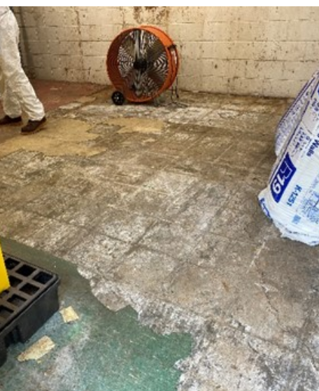
Broken vinyl floor tile poses severe health risk. Only specialized workers with appropriate PPE may enter the building until asbestos abatement has been conducted.
