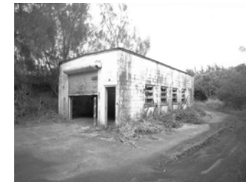
warhead building where missiles were assembled
