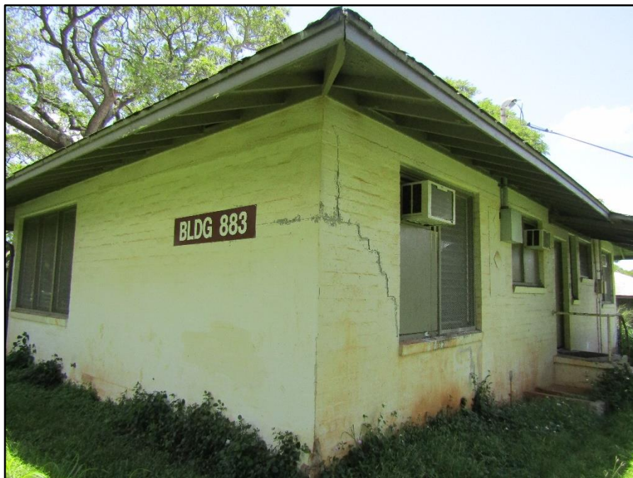
Bldg 842 (marked as Bldg 883)- Cracks near the north end of west wall, under window sill to corner.
