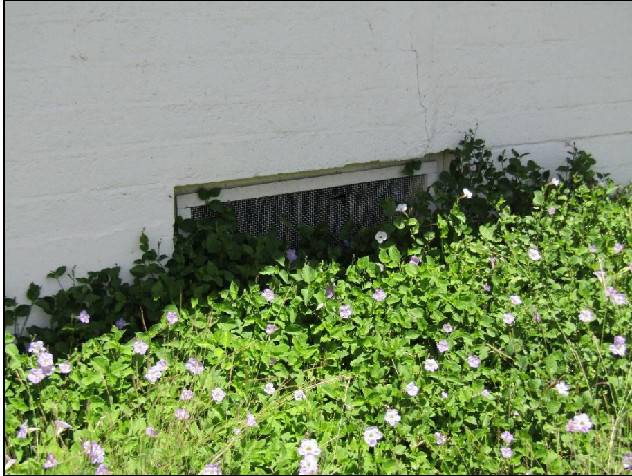
Bldg 827 (Bldg 878) - Screened foundation vent at rear.
