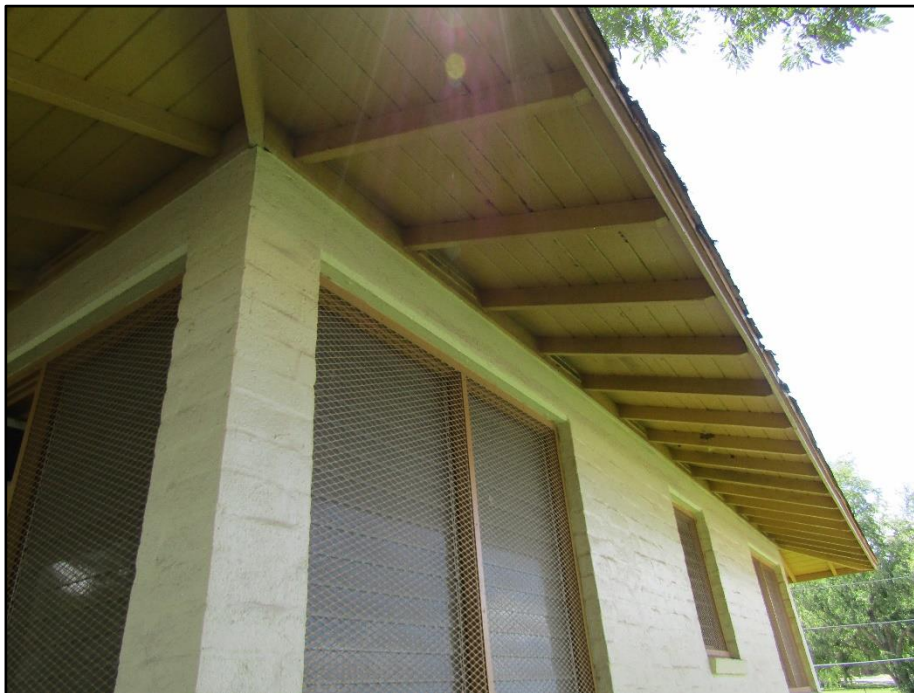
Bldg 827 (Bldg 878) - Overhanging eaves with eave vents.
