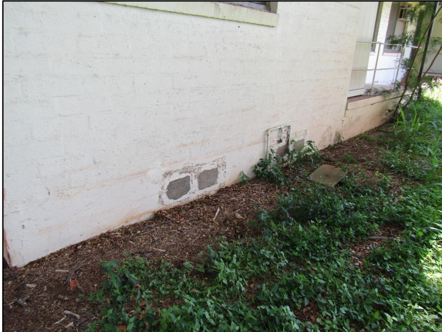
Bldg 826 (Bldg 877) - Close-up of concrete infilled foundation vents at front.
