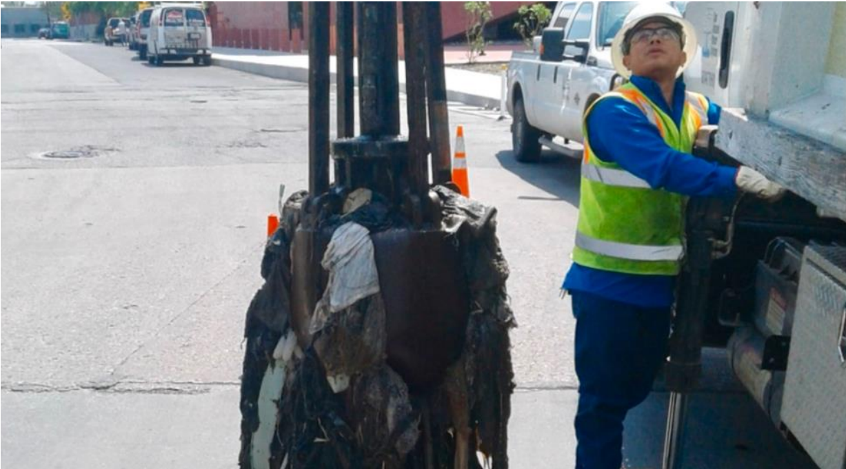
Photo Courtesy of San Antonio Water System
