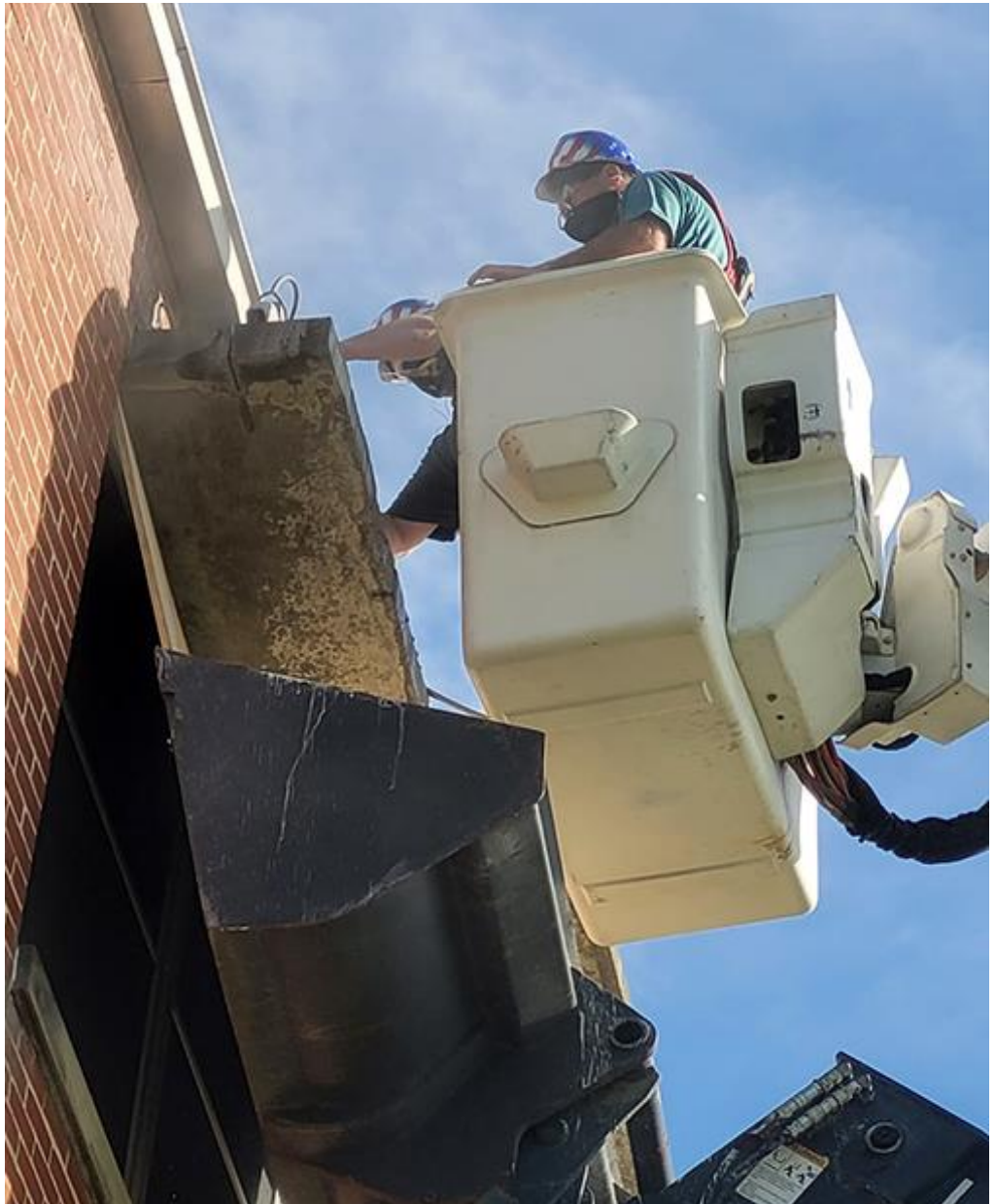
The DPW team proactively addressed a critical safety concern at the home of U.S. Army Medical Materiel Development Activity by repairing a crumbling concrete awning on the building's exterior. (Photo courtesy of Installation Safety Office)
