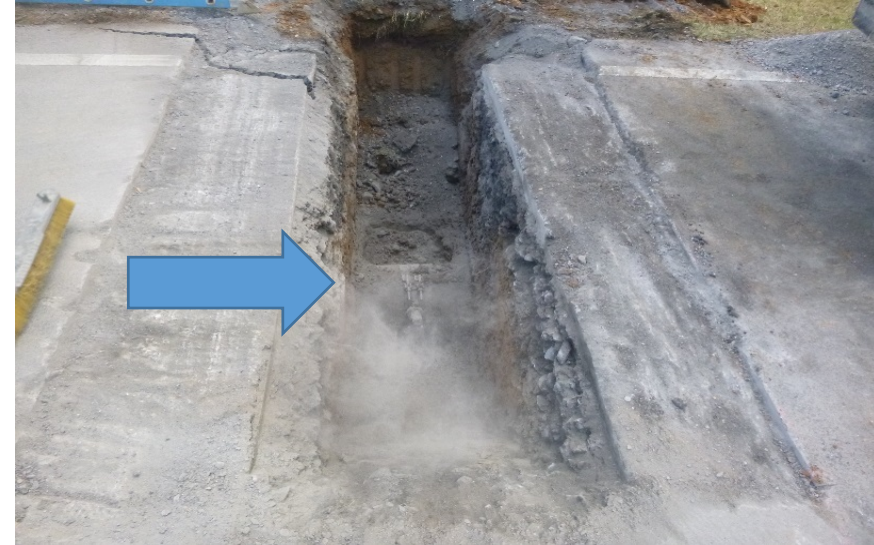
Kemp Lane road cut and exposed water main.
