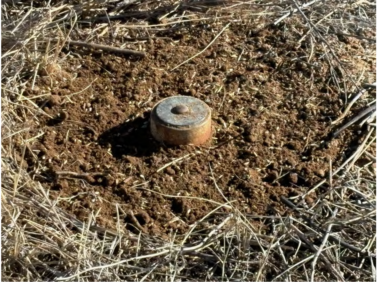
The repaired area at ER76 seeded.
