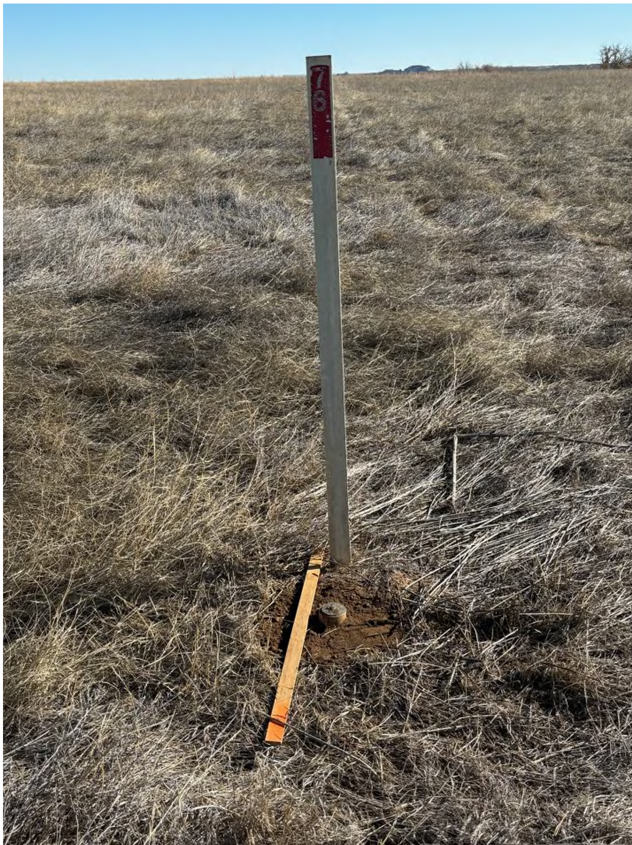
The north side of the repair at ER76.
