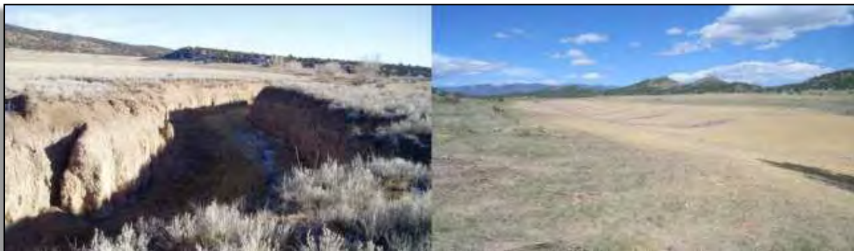
Bank sloping before and after
