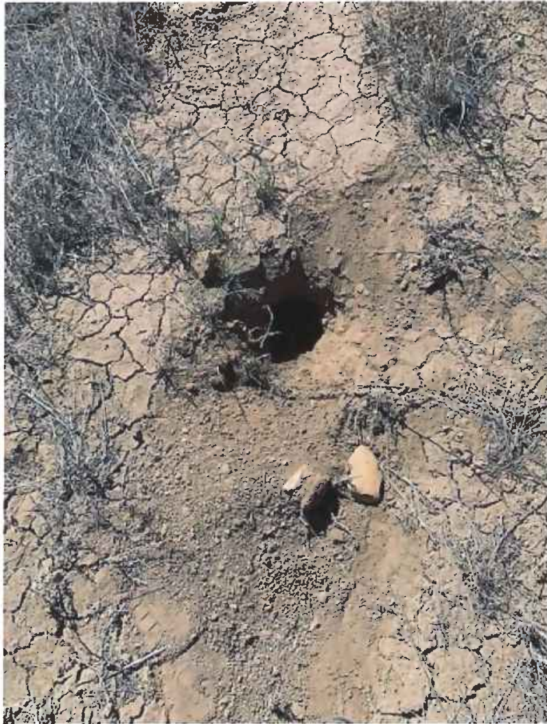
Hole observed along the perimeter channel at the ELF and backfilled using existing soil.
