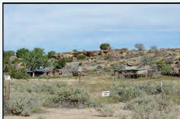
Protection Fences with Restricted Access Signs
