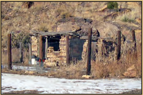
Stone structure with hand cut juniper vigas and latillas built around 1891. Possibly a residence later modified into a chicken coop.
