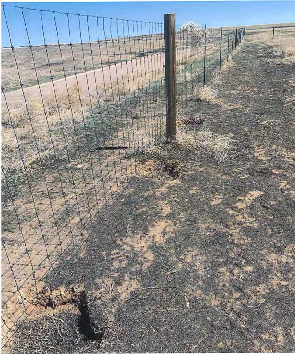
Photo 6 Sinkholes under perimeter fence
