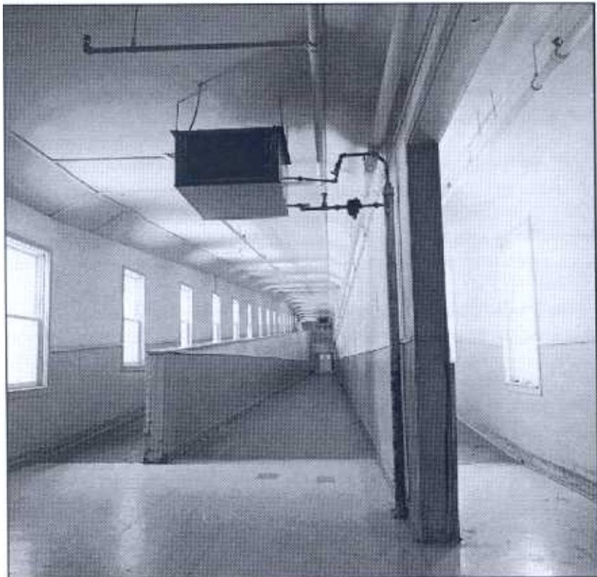
Figure 17. Interior shot of ramp system and double corridor connecting Building S6251 to the hospital complex. The system of covered walkways united the entire complex. The ramp system allowed wheelchairs, gurneys, and supply trolleys to move easily between buildings and floors.
