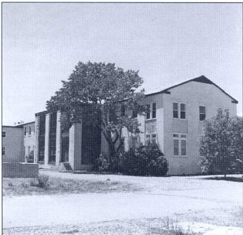
Figure 10. View of a neuropsychiatric ward (Building S6253) showing screened porches accessed from the common-ward rooms.
